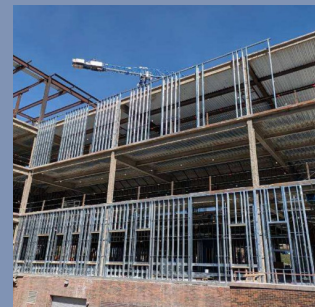
Exterior wall framing continues around the south half of the building.
