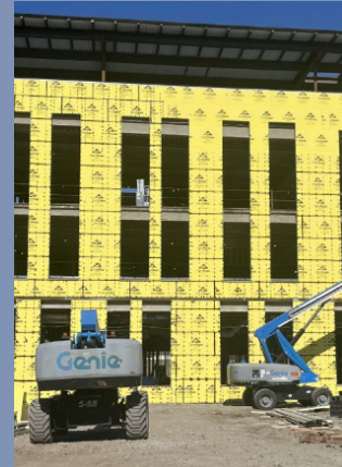
Crews are installing sheathing material at the Southeast wall elevation.
